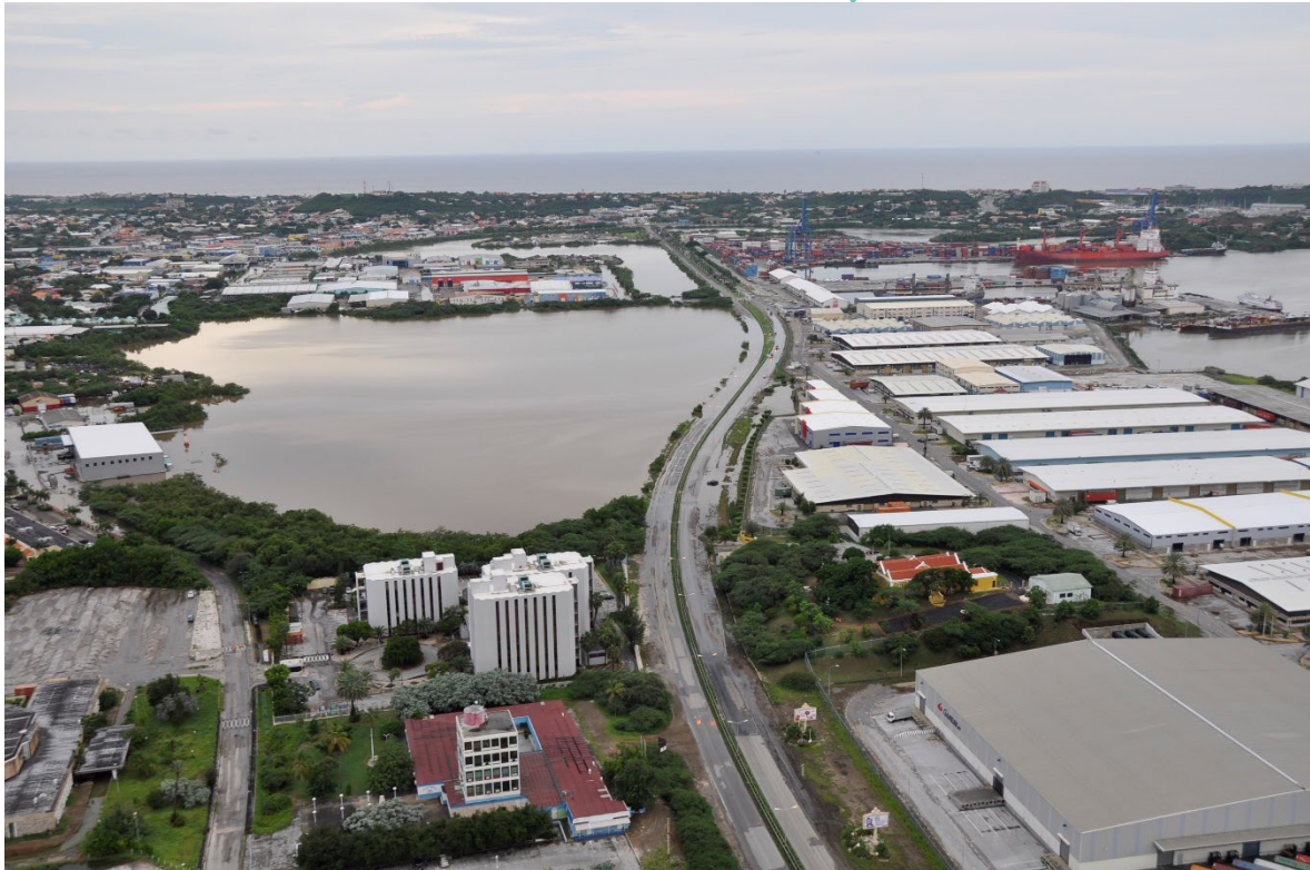
Figure 12: An image of floods caused by Tomás in November 2010.
